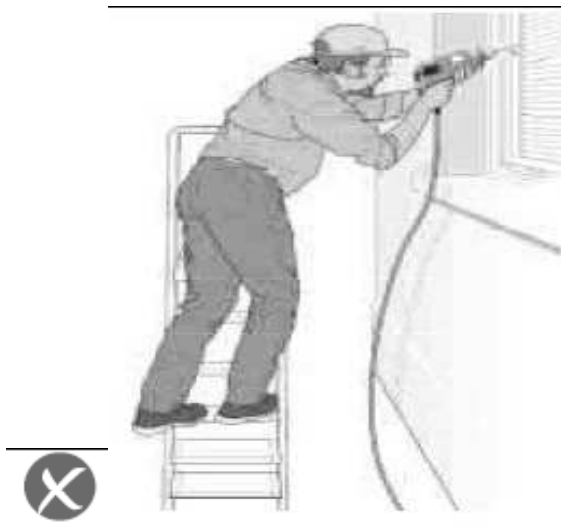
Incorrect – steps side on to work activity
