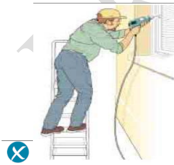
Incorrect – steps side on to work activity
