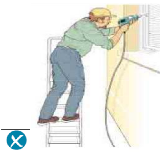
Incorrect – steps side on to work activity
