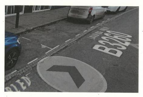
The bricks in the crossing near the Plume of Feathers sunk badly last year and were removed for safety reasons. The bricks in the crossing by the White Hart are now starting to sink and will need attention in due course. I
