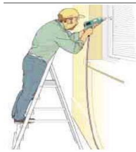
Correct – steps facing work activity
