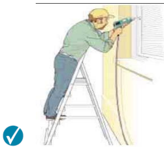
Correct – steps facing work activity
