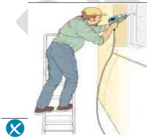
Incorrect – steps side on to work activity
