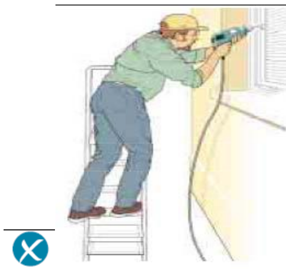
Incorrect – steps side on to work activity
