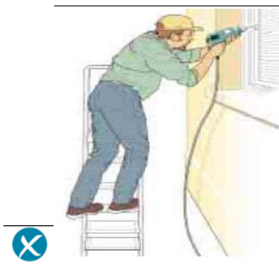
Incorrect – steps side on to work activity
